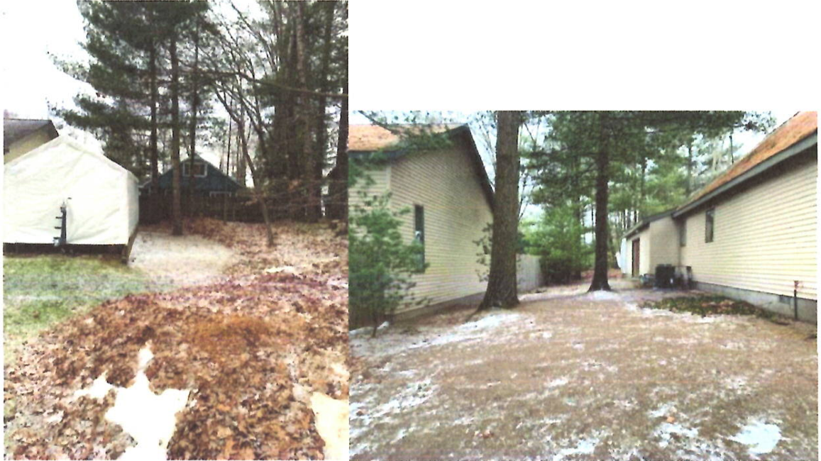
Left picture: Rear property line along with cover for boat. Right picture: the north side of the parcel with the house on the right and the building on the left being a neighbor's building a couple of feet on the parcel.
